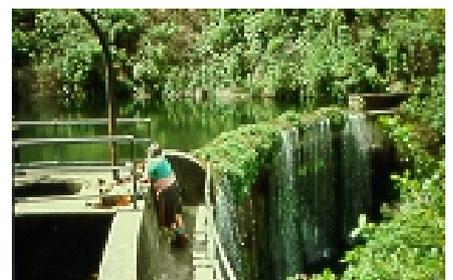
The dam operated until the Kaitoke Scheme commenced supply in 1954. The dam continues to retain a lake, however the volume of the dam has decreased over the years because of silting. In 1988 the dam was drained and silt was measured to 6.3 metres below the spillway. Eels and some brook trout now inhabit the lake.
