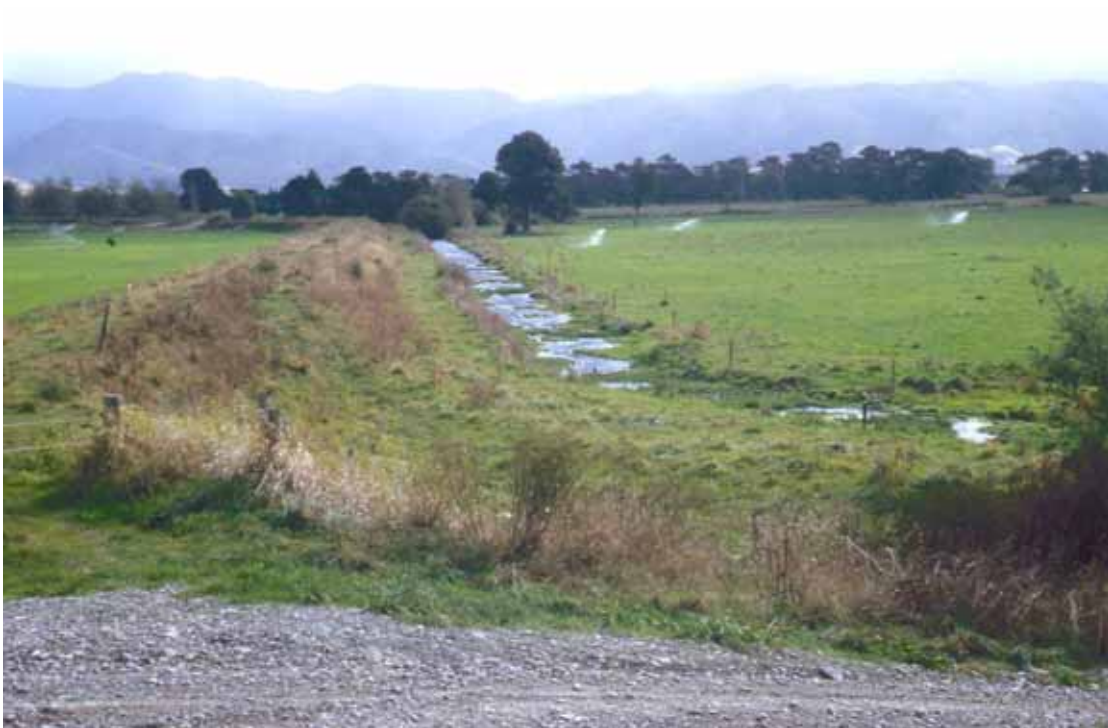
Photo 3.8.2: Tauherenikau Seepage Drain near its source from under the river stopbank. Barton's Lagoon ca 2km far left. Note extensive use of irrigation.
