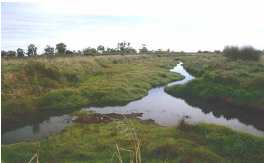
Photo 8.6: Confluence of the two collecting streams from the southern drainage network. Water flows into the drainage lagoon beyond. Note considerable rise to the wetland on the left.
