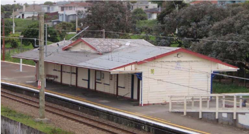
Tawa Station before demolition
