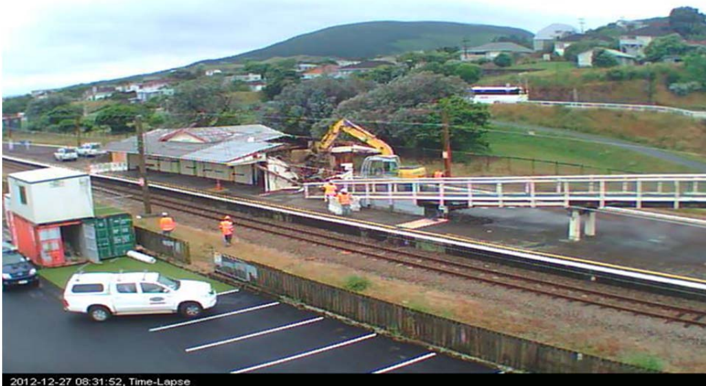
Tawa Station Demolition in progress
