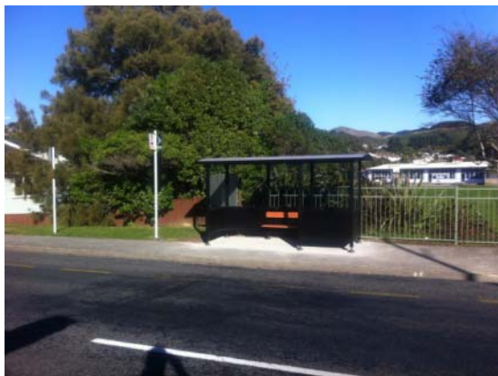
Shelter replacement Mungavin Avenue, Porirua
