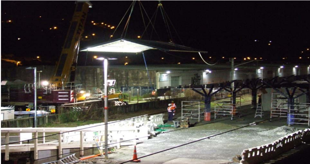
The new Tawa Station roof being moved into position
