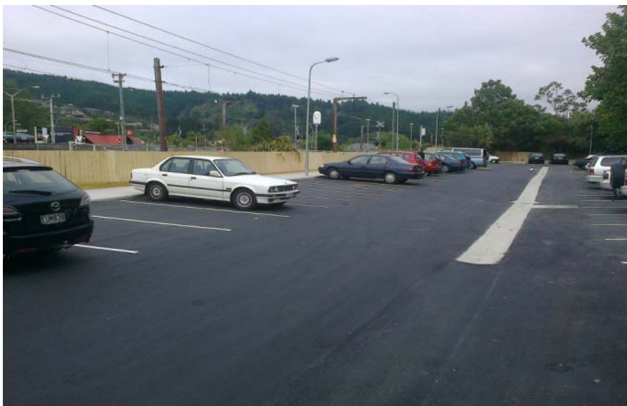
Silverstream post reconstruction
