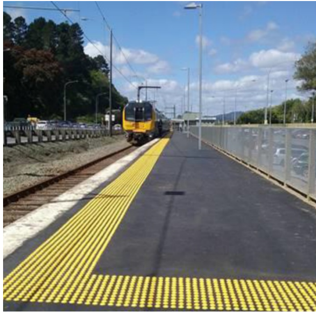
Melling platform resurfacing and new fence.
