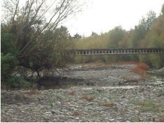
Figure 3: Private vehicular bridge (XS38)
