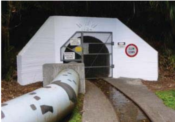
The three kilometre long Orongorongo Tunnel provides access for water pipeline inspections and maintenance. It runs from the Big Huia Creek Intake in the Orongorongo Catchment through to the George Creek area of the Wainuiomata catchment. A diesel engine and cart carry gear and equipment. Glow worms live in the tunnel and can be seen approximately 30m from the tunnel entrance.
