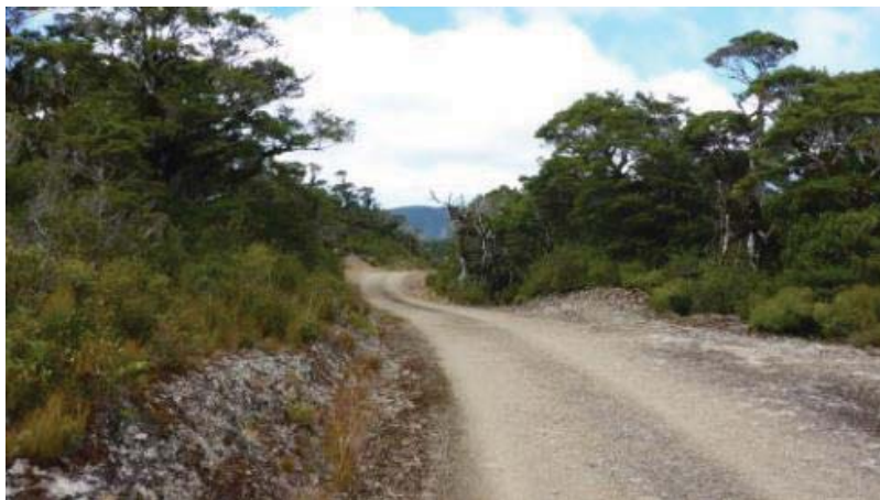
Orongorongo road is a key asset providing management access into the remote Orongorongo water catchment. Following a ridge line, it
