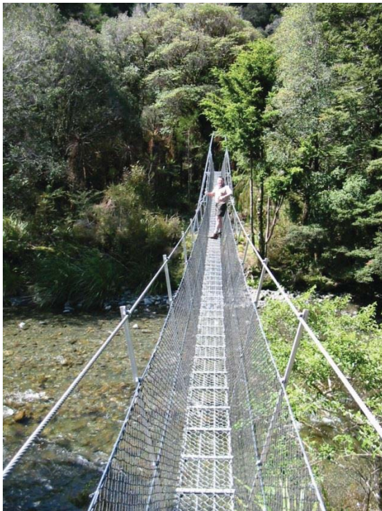
A suspension bridge at Hutt Forks minimises risks from water contamination via river crossings and provides access to the Quoin Ridge route
