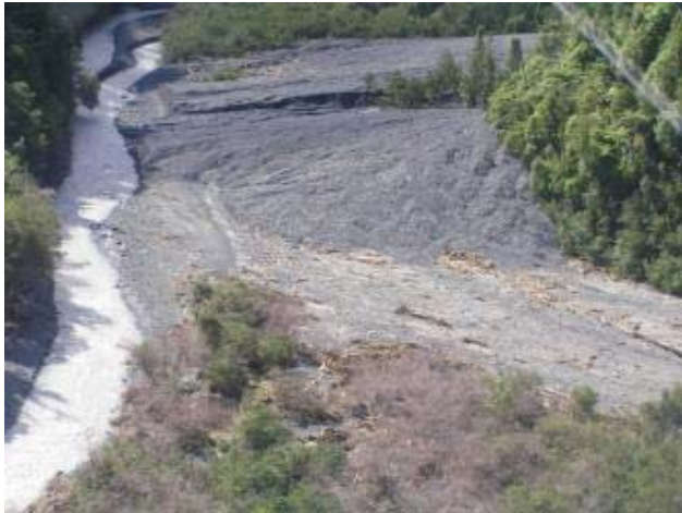
River bank and asset protection measures such as gabion rock baskets are utilised as flood and erosion stabilisation measures
