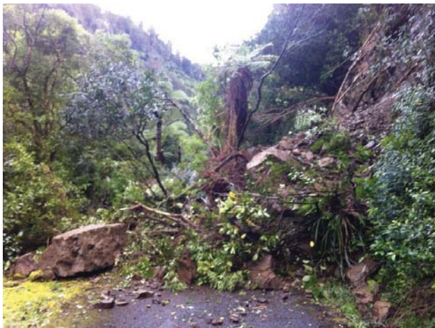
Rock slip covering the access road to the weir at Kaitoke after heavy rain, August 2016
