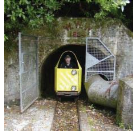
The three kilometre long Orongorongo Tunnel provides access for water pipeline inspections and maintenance. It runs from the Big Huia Creek Intake in the Orongorongo Catchment through to the George Creek area of the Wainuiomata catchment. A diesel engine and cart carry gear and equipment. Glow worms live in the tunnel and can be seen approximately 30m from the tunnel entrance.
