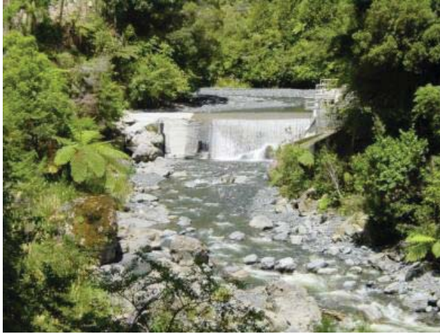
Orongorongo Weir and water intake, Orongorongo River. Assets such as weirs are being progressively seismically strengthened via asset renewal programmes.
