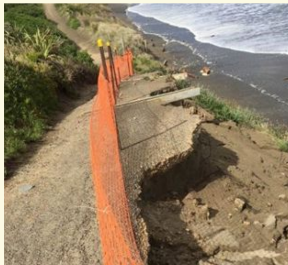
QEP coastal track after February 2018 storm. More frequent and severe storms as part of climate change means that the coastal track will progressively move inland where its less susceptible to damage.
