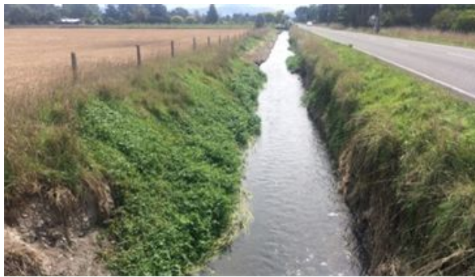
Manaia roadside drain after spraying and clearing of flood debris
