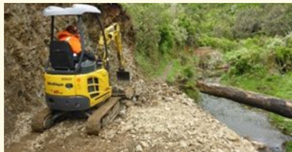
Flood damage repairs to the Korokoro Dam track provided the opportunity to improve the track and make it more resilient to future flood events.
