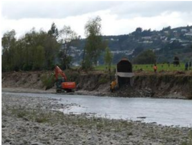
Hutt River Edge Protection works - Taita Berms
