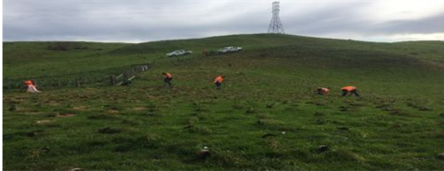
Transmission Gully planting contractors at work
