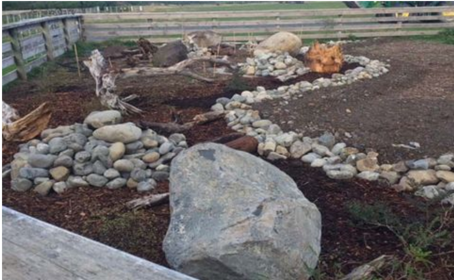
Lizard garden under construction
