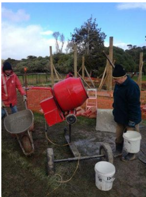
Dell Picnic Shelter construction
