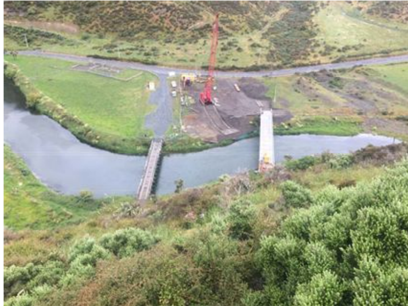
Baring Head bridge construction
