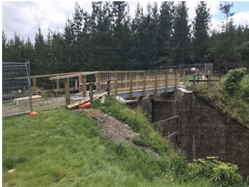
Martins #1 bridge – in construction
