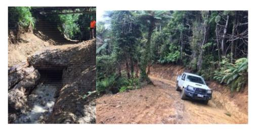
Culvert installation in progress below Perhams Road Bailey Bridge. Pram Track Upgrade
