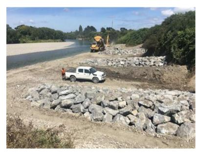
Photo 5: Dakins Road completed rock groyne construction.
