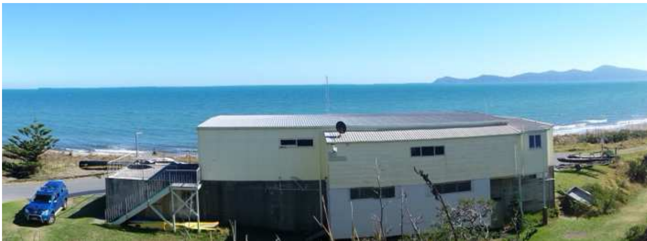
Figure 14 - Rear view of the current building
