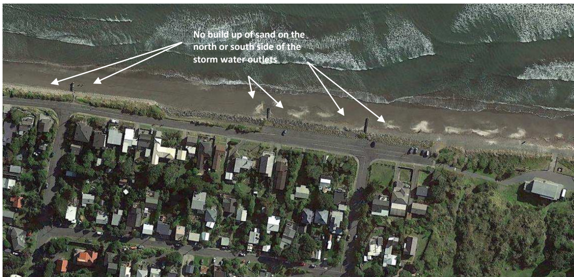
Figure 4: Lack of sand deposition around storm water outlets
