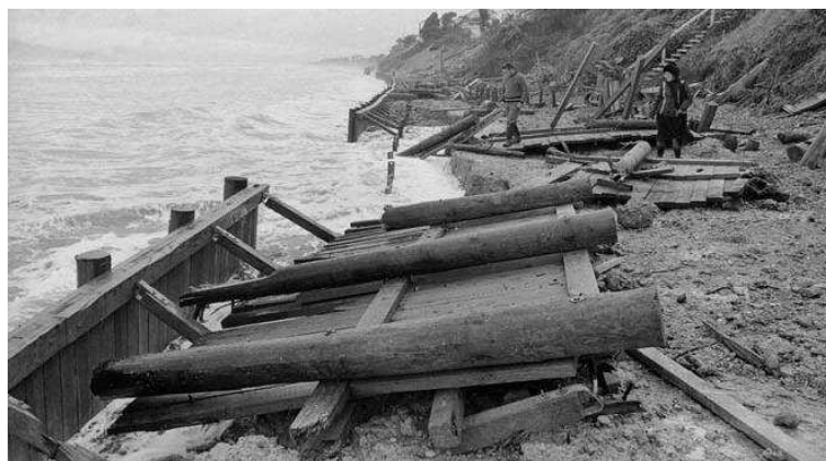
Figure 5: Storm damage at Paekākāriki 1978
