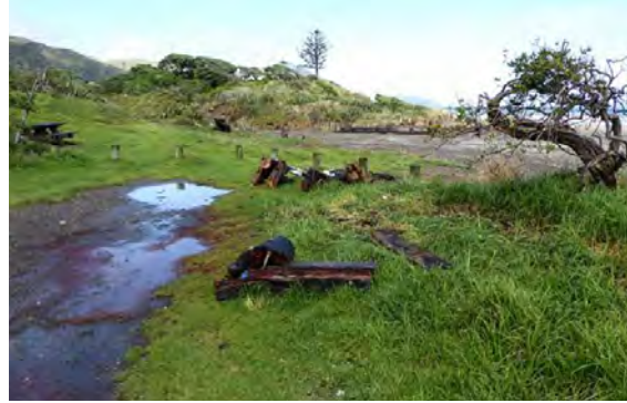
Debris from footbridge scattered around Wainui Stream mouth
