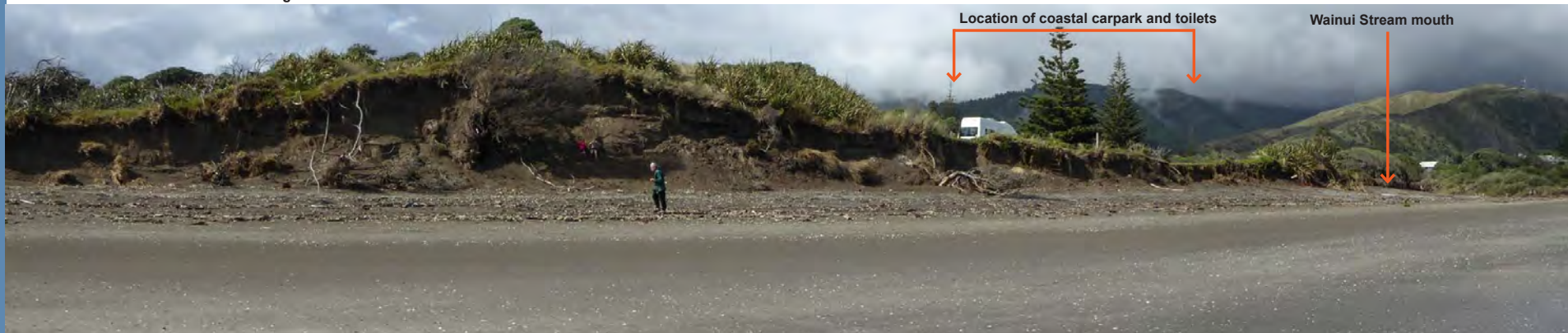
Erosion north of Wainui Stream reducing beach access
