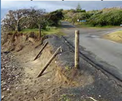
Coastal ring road eroding after storm surges
