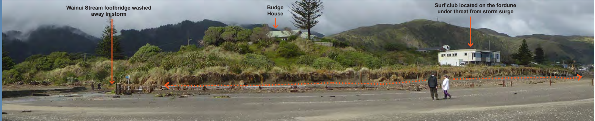
Erosion at beach edge in front of surf club
