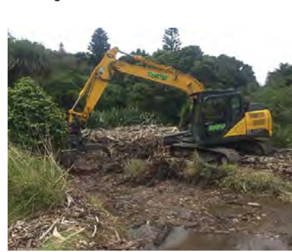
Clearing debris from the stream after storm 2018
