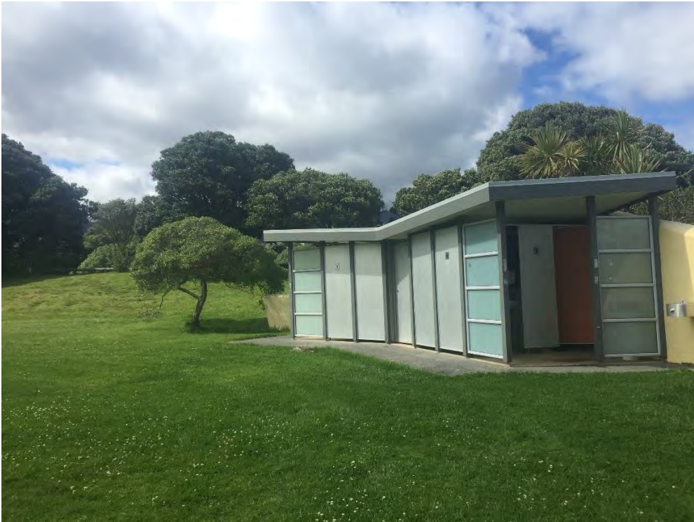
Plate 10: An existing toilet block at Queen Elizabeth Park. 19 November 2020.
