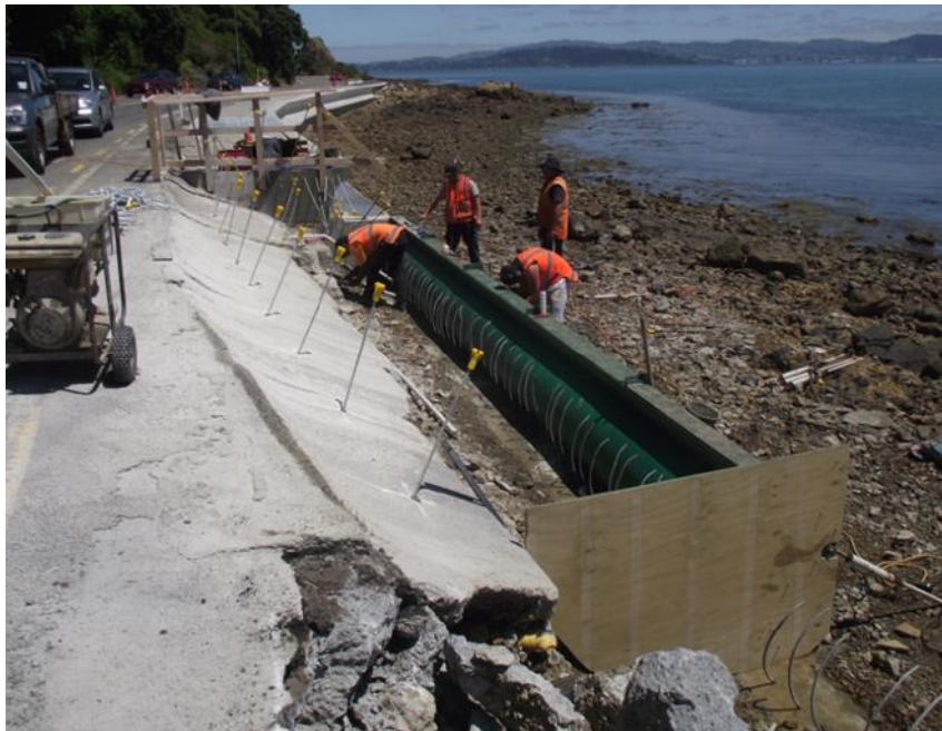
Figure 11: Example of in situ construction methodology at York Bay.
