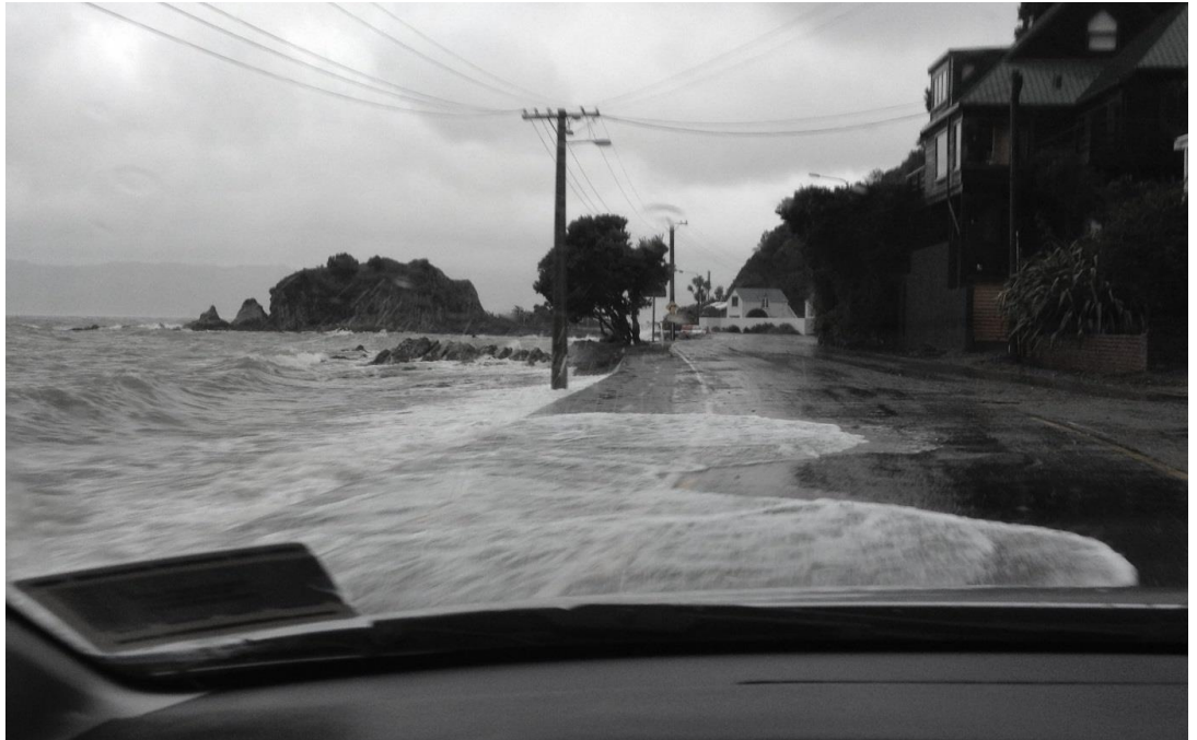
Figure 6: Wave overtopping at Mahina Bay (22 June 2013) 3
