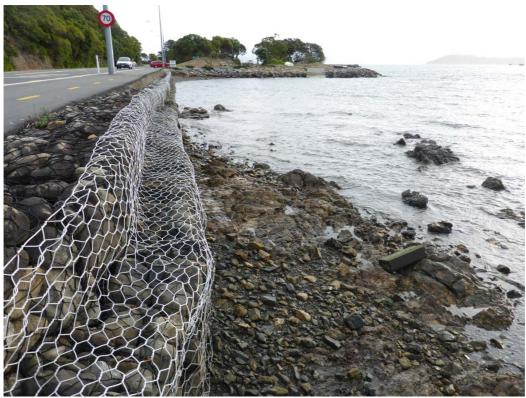
Gabion baskets in southern Lowry Bay Figure 11 Example of existing seawall type: gabion baskets.
