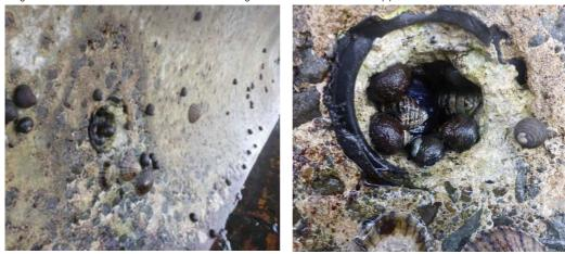
A weep hole in the surface of the existing new curved seawall at York Bay provides additional refuge areas for taxa when the tide is out.
