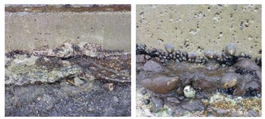
Larger substrate embedded in the toe of the existing new curved wall at York Bay provides additional habitat for biota.
