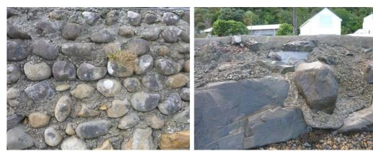
Concrete-aggregate wall with large cobbles set in place with concrete at Sorrento Bay
