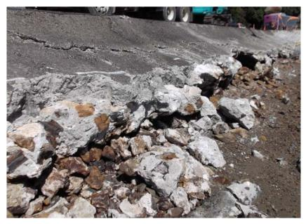
Figure 4-1: Removal of sections of existing seawall
