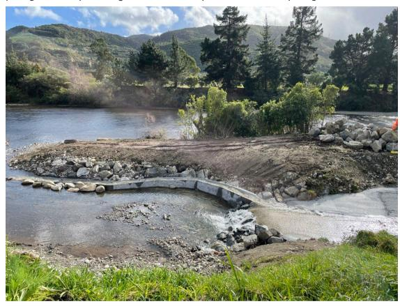
Figure 5: Site 1 - Stokes Valley Stream fish passage and repaired weir
